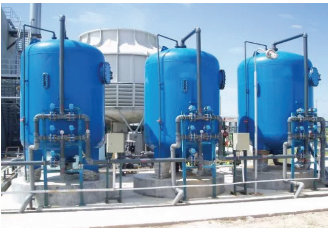
Capacity: 30\text{m}^3/\text{hr} ~ 150\text{m}^3/\text{hr} (Ms Vessel)
