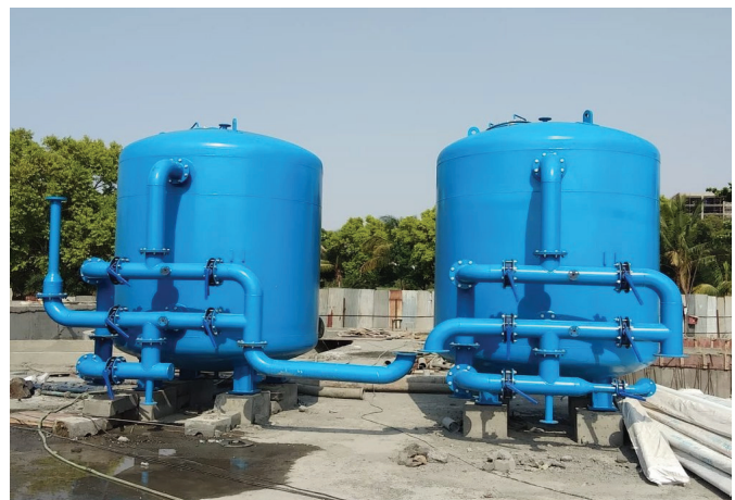
Capacity: 20\text{m}^3/\text{hr} ~ 50\text{m}^3/\text{hr} (Ms Vessel)
