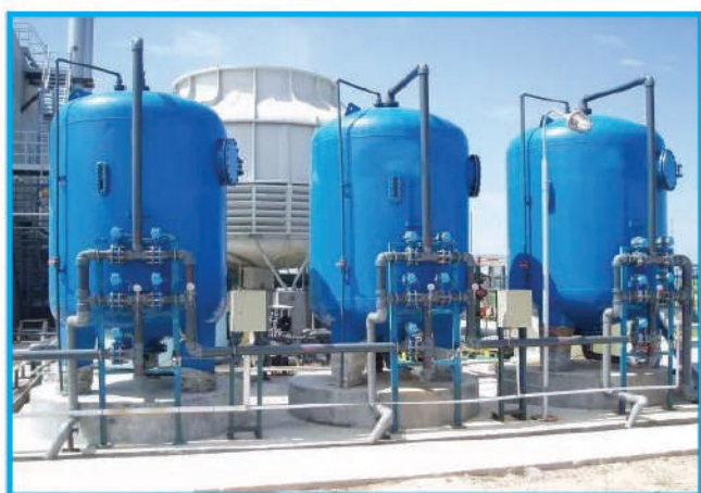
Capacity: 30\text{m}^3/\text{hr} \sim 150\text{m}^3/\text{hr} (Ms Vessel)
