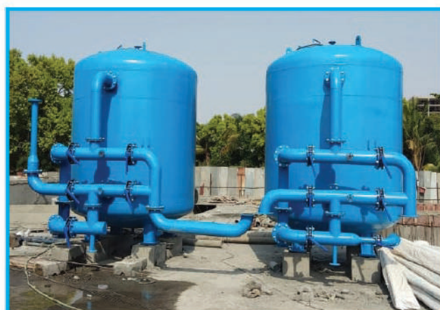
Capacity: 20\text{m}^3/\text{hr} \sim 50\text{m}^3/\text{hr} (Ms Vessel)
